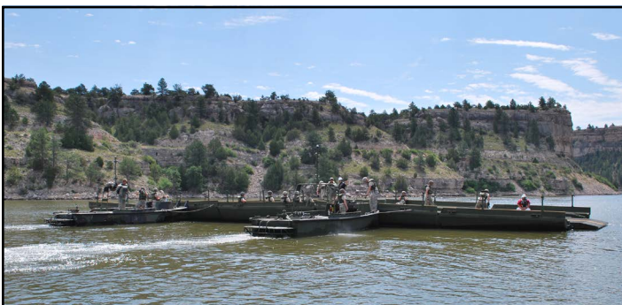
Soldiers with the 1041st Engineer Company, Wyoming Army National Guard, begin the process of connecting bays of the Improved Ribbon Bridge, or IRB, July 21, 2010 at the Guernsey Reservoir, in Wyoming. The Soldiers work under the supervision of civilian instructors from AM General, the bridge's manufacturer. The IRB replaces the Standard Ribbon Bridge, developed in the 1970s. The bridge, which can be turned into a raft, can carry a heavy equipment transport loaded with an M1A2 Abrams tank. The 1041st is based in armories in the Wyoming cities of Rock Springs, Evanston and Afton. (U.S. Army file photo/2nd Lt. Christian Venhuizen)
