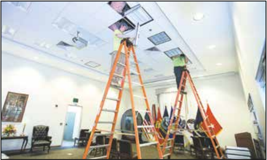
Tim Dworshak and Brian Gier, both lighting retro fitters, replace old light fixtures with new high energy efficient LED fixtures March 8 in building 39 on the Fort McNair portion of Joint Base Myer-Henderson Hall. The conversion will cost $170,000 and is expected to save 35,000 kilowatts of electricity, as well as $3,500, per year.
