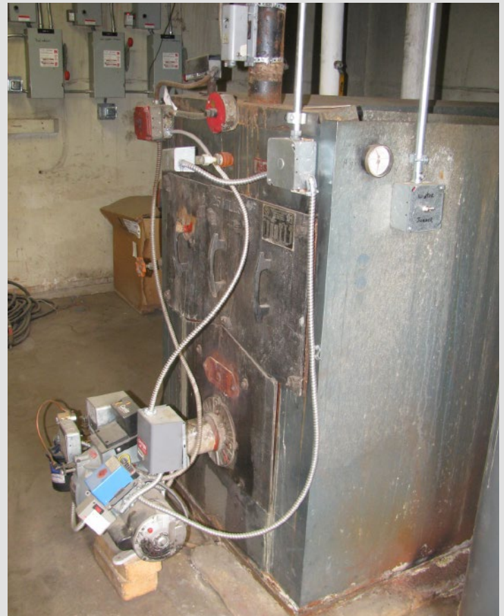
Old fuel oil boiler that burned 11 gallons per hour.
