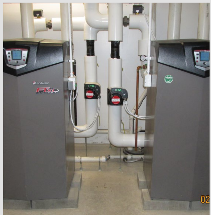
New high efficient gas boilers that burn between 1.5 to 3 gallons of fuel oil equivalent an hour each.
