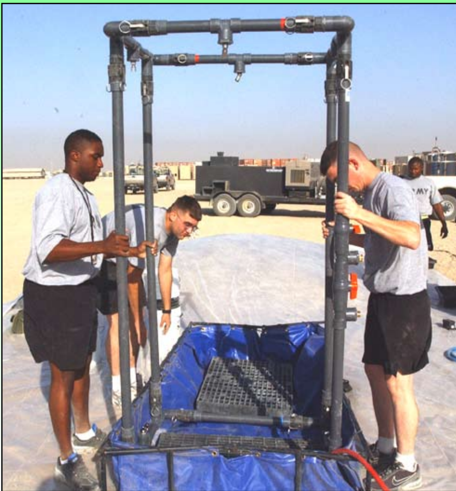
44th Chemical Company Soldiers set up a mobile shower system during a training exercise at Camp Arifjan, Kuwait, Nov. 9. The shower is used during the decontamination process.
