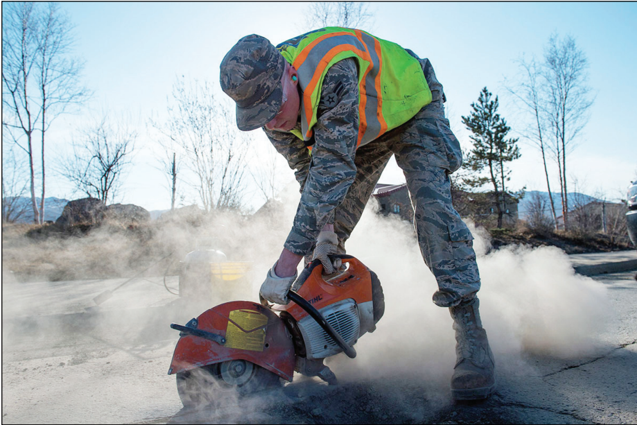
ABOVE: Airman 1st Class Jeremy Clapham, assigned to the 773rd Civil Engineer Squadron, uses a saw to cut into the asphalt around a pothole while performing road improvements on Joint Base Elmendorf-Richardson last April. The 773rd CES Airmen repaired potholes around base to maintain safe road conditions. (U.S. Air Force photo/Alejandro Pena) LEFT: Airman 1st Class Michael Ramseur, 773d Civil Engineer Squadron structures apprentice, signals traffic on Provider Drive while 773d CES personnel repaint lines in 2014. Alaska’s weather is tough on roads, necessitating frequent repair.— (U.S. Air Force photo/Airman 1st Class Tammie Ramsouer)
