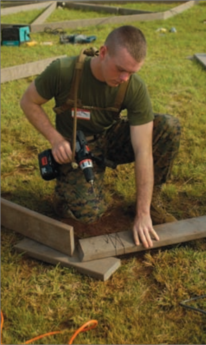
Drilling holes into recycled plastic lumber, Pfc. Travis Surls, rifleman, 1st Battalion, 3rd Marine Regiment, helps construct a frame for one of the larger playground structures. Volunteers made frames for playground equipment shaped in Hawaiian designs suggested by students. New additions to the playground include a gecko-shaped slide, twin palm treehouses and a turtle-shaped stage.
