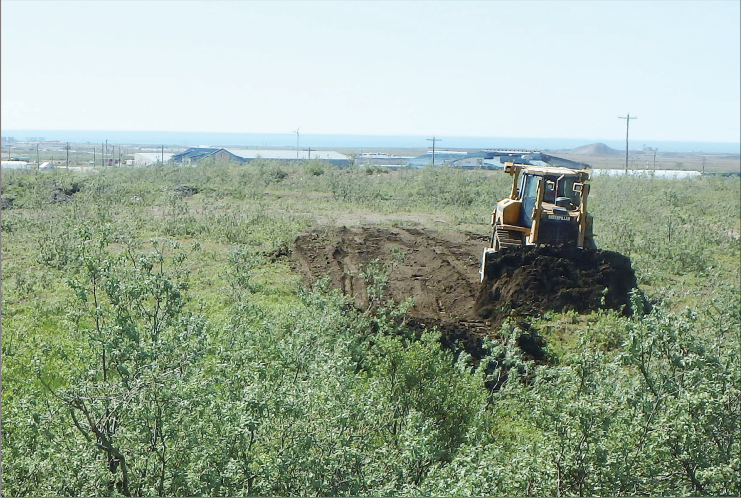
A dozer begins grading a landfarming cell near the Tank Site E project near Nome, Alaska. Landfarming is a potential solution to meet the needs of the U.S. Army Corps of Engineers – Alaska District’s Formerly Used Defense Sites program across Alaska. The process includes removing contaminated soil from the source location, spreading it across an expansive area one to two feet thick, tilling consistently and then letting nature take control to degrade the pollutants. The Tank E site is where a World War II-era fuel storage tank, containing up to a million gallons of diesel fuel, had deteriorated. The Corps removed the tank and its foundation, and is now cleaning up about 30,000 tons of contaminated soil. (Courtesy photo/U.S. Army Corps of Engineers)
