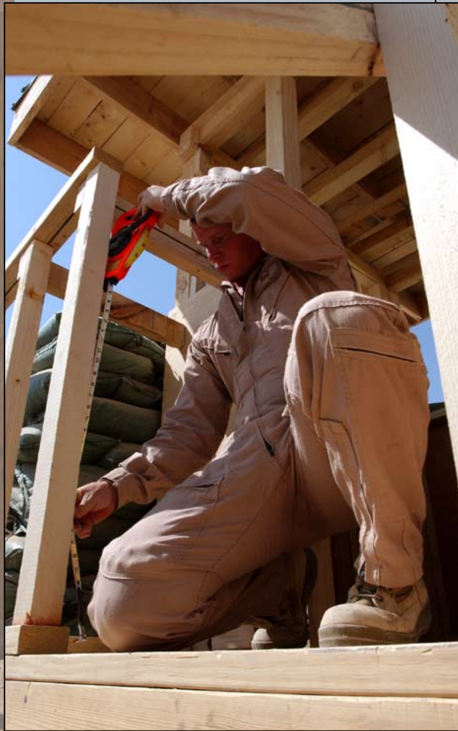
Marine Cpl. Christopher Perry, 3rd Battalion, 8th Marine Regiment, 22nd Marine Expeditionary Unit (SOC), a native of Hughes Spring, Texas, measures the baluster at the top of the stairs to place a railing on the watch tower dubbed FOB Semper Fi in the Training Village on Camp Buehring, Kuwait, Sep. 29.
