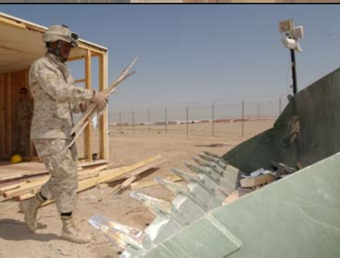
Cpl. Joan Jimenez, a backhoe operator with 3rd Battalion, 8th Marine Regiment, 22nd Marine Expeditionary Unit (SOC), and a native of Dominican Republic, loads trash and broken boards into the loader of a backhoe at the dismantled IED Lane in the Training Village at Camp Buehring, Kuwait, Sept. 29.
