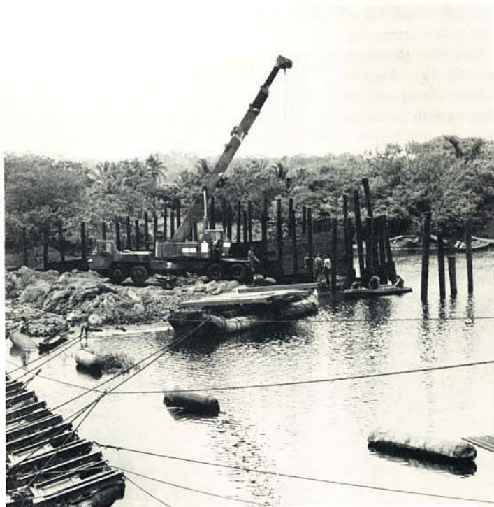
Alabama Army Reserve engineers built a permanent bridge linking Gobeia to civilization on Panama's Atlantic Coast.
