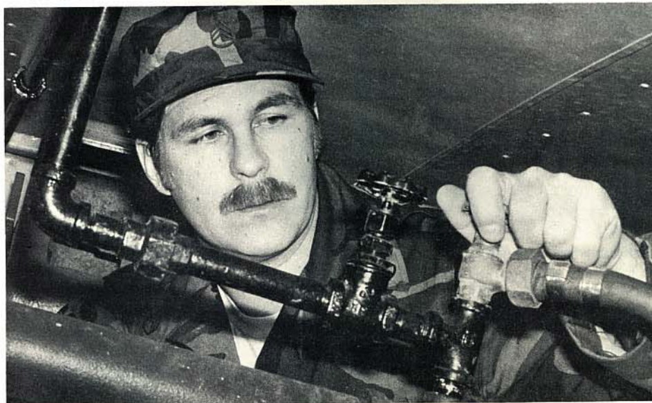
SSgt. Gary Byron is shown here working on the water purification system for the 286th Engineers.
