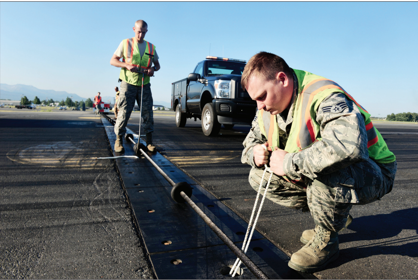
Robert Gordon, a power production journeyman with the 773d Civil Engineering Squadron, ties one of the ropes which help hold the cable for the BAK-12 aircraft arresting system in place on the runway. The BAK-12s on Joint Base Elmendorf-Richardson are designed to bring out-of-control aircraft to a safe stop with minimal damage. (U.S. Air Force photo/Airman 1st Class Kyle Johnson)
