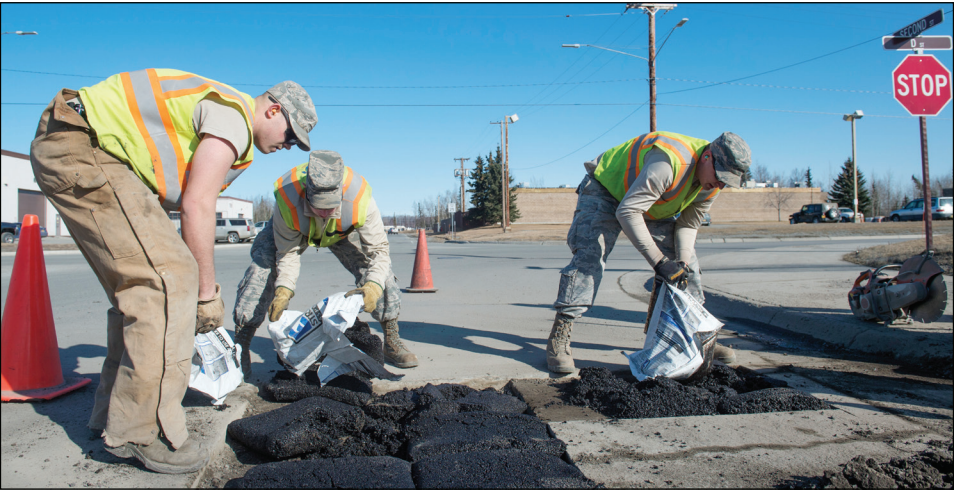
Airmen improve JBER roads April 3. Pothole repair is a never-ending task in Alaska. (U.S. Air Force photo/Alejandro Pena)
