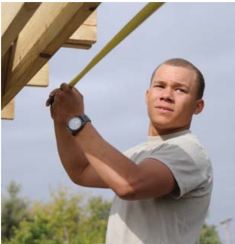
Airman 1st Class Marcus Rhodeman, 184th Security Forces Squadron, measures for correct spacing between boards while building a pergola.
