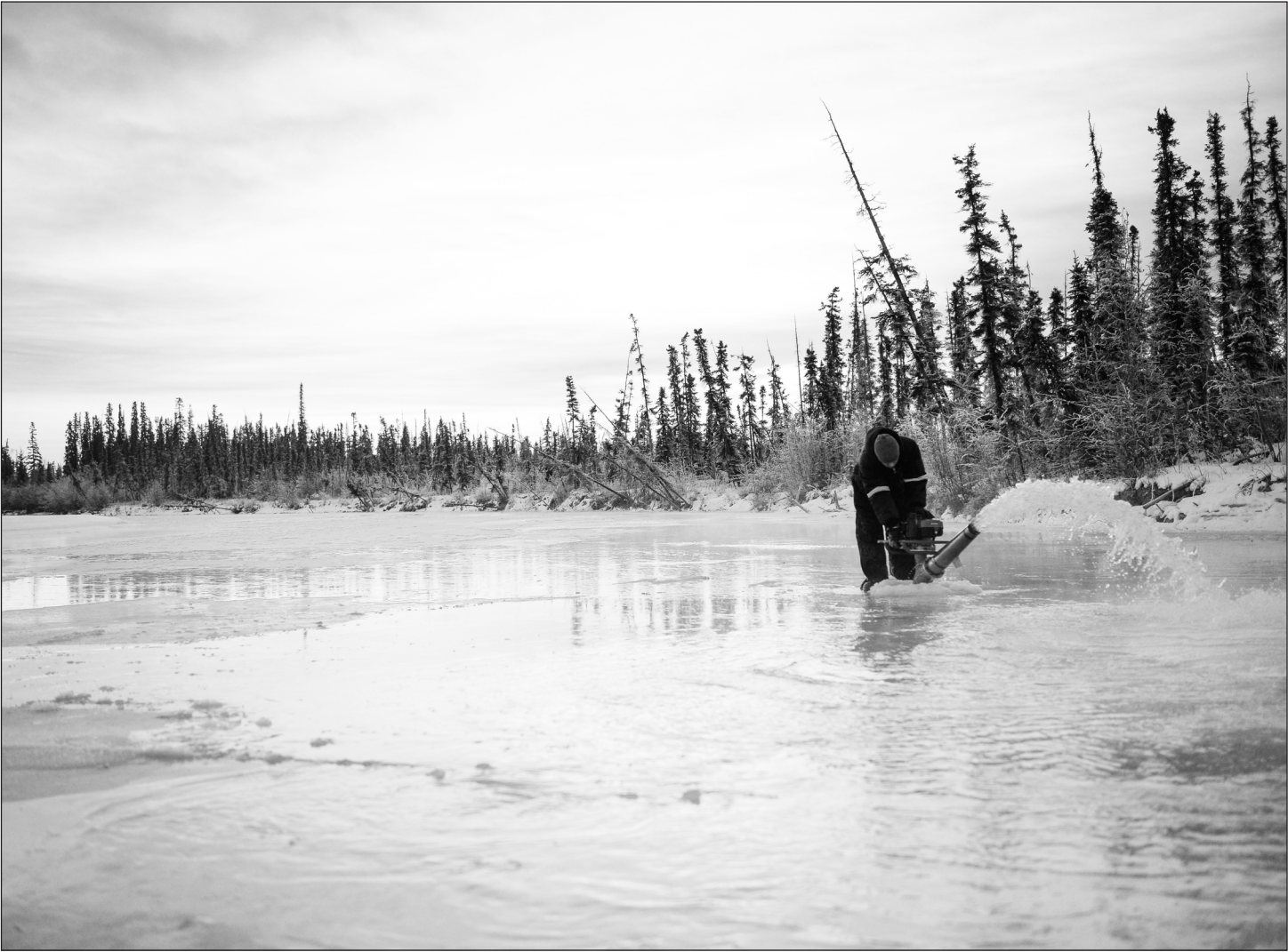
Senior Airman Jerry Mitchell, a heavy-equipment operator assigned to the 354th Civil Engineer Squadron, uses a water pump while constructing an ice bridge in Fairbanks in November. The bridge must be constructed every other year to provide access to the $20 million range complex used to train pilots from around the world during Red Flag-Alaska exercises. (U.S. Air Force photo/Staff Sgt. Shawn Nickel)
