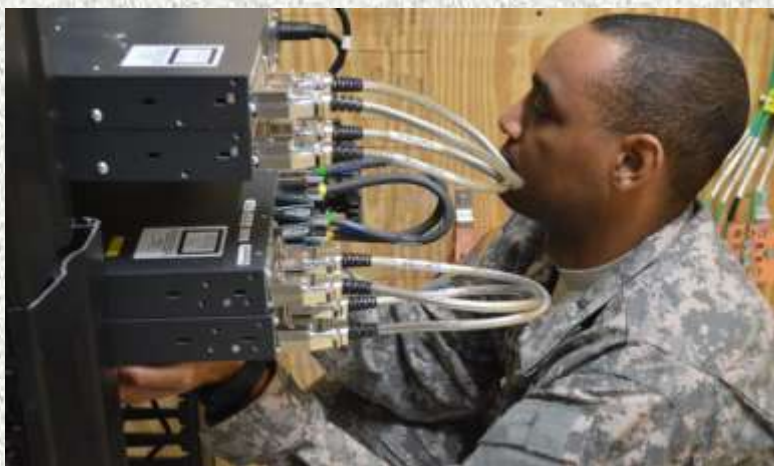
Signal Soldiers installing new switches as part of the I3MP upgrades
