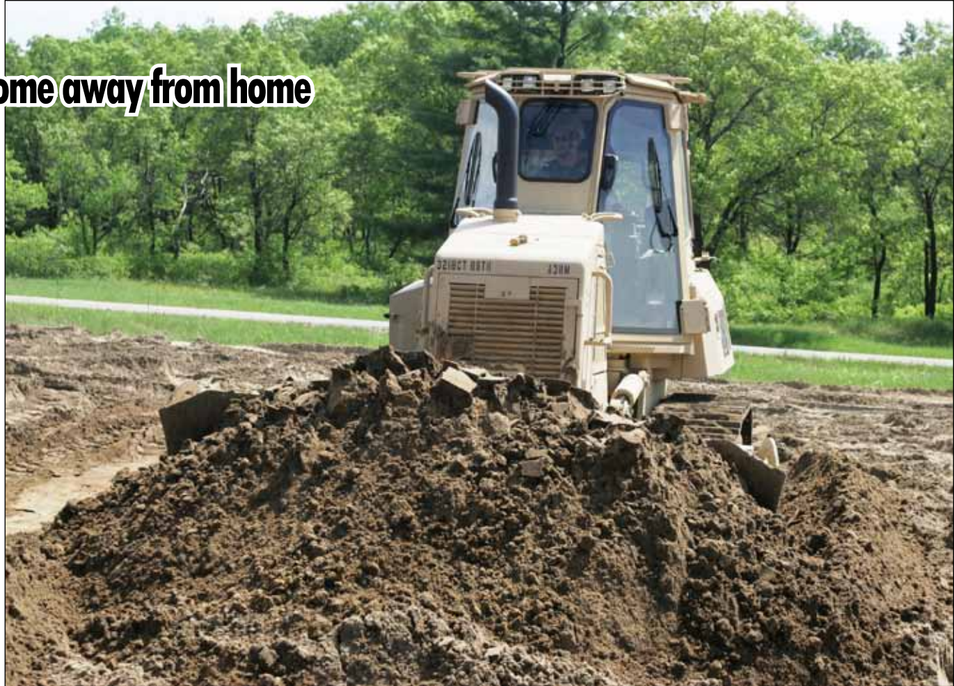
A combat engineering Soldier with Company A, 32nd Brigade Special Troops Battalion, a Wisconsin National Guard unit in Onalaska, uses a bulldozer to build an earthen berm for a training forward operating base on Fort McCoy's North Post. Fort McCoy Public Affairs photo by Scott T. Sturkol
