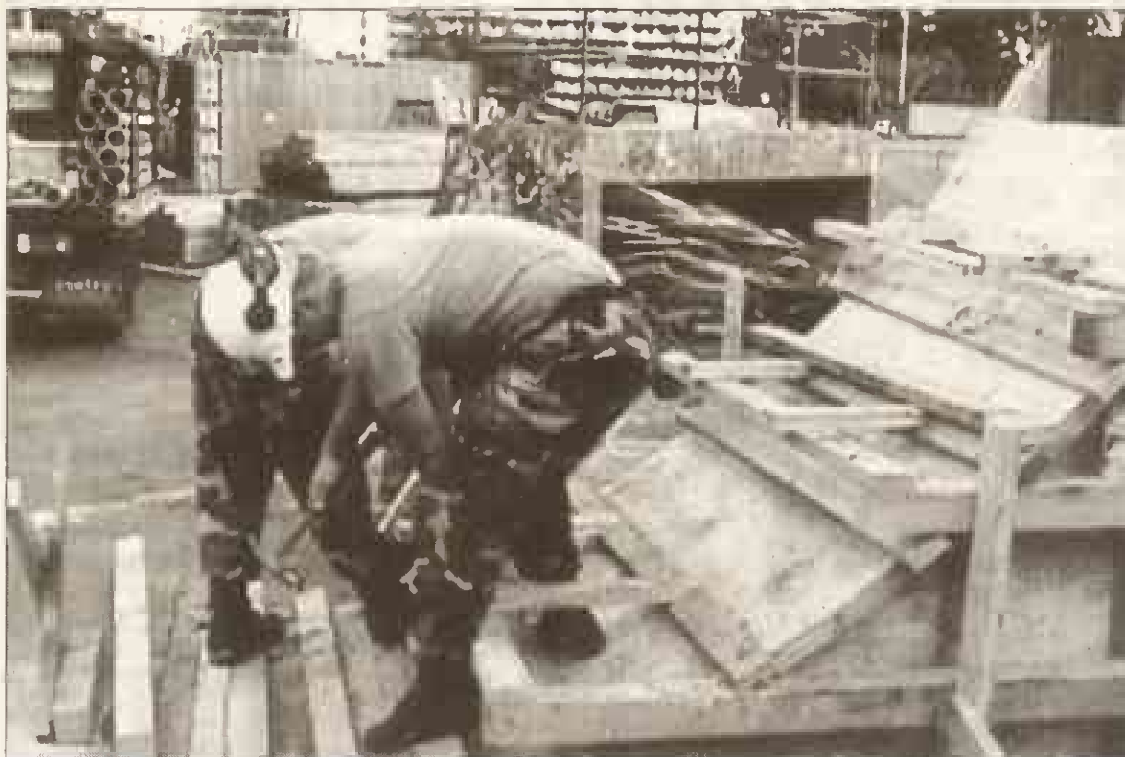
Photo courtesy of the 84th Engineer Battalion Pfc. Leonard Wdowik from Company A, 84th Engineer Battalion, hammers together framework for one of the obstacles before concrete is poured.
