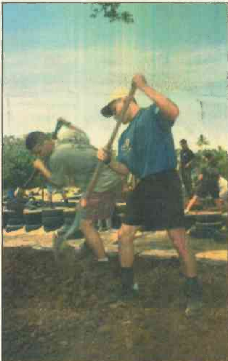
SSgt. Stephen Guide LCpls. Jacob Grahman, left, and Shane Roushar, B Company, 1st Battalion, 3d Marines, cover tires with dirt while volunteering to help Akahi Elementary School in Kailua build a new playground. Marines from A Co., 1/3 helped Saturday, while 24 other volunteers from B Co. came out Sunday.
