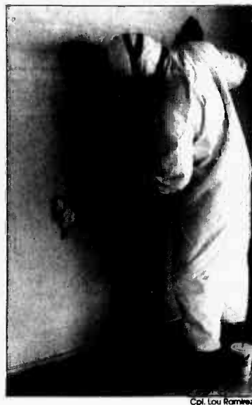
Paint Contractors protect themselves from lead particles that may be in the air when paint is removed.
