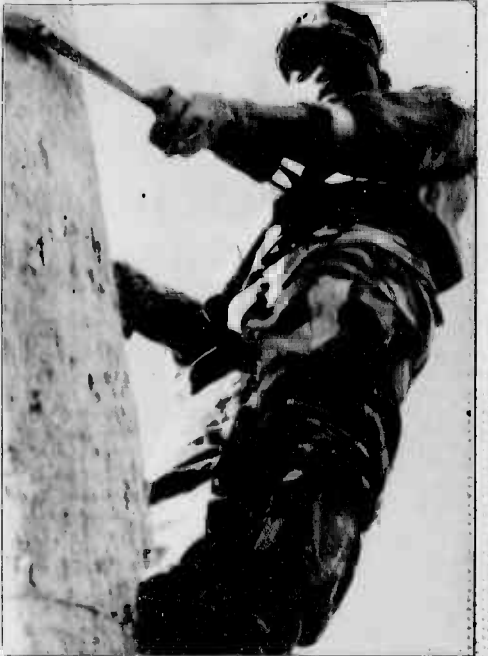
LCpl. William Patterson, a field wireman with B Co., 7th Communication Bn., climbs a pole using a safety belt and gaff set. This gear is essential for the field wireman.
