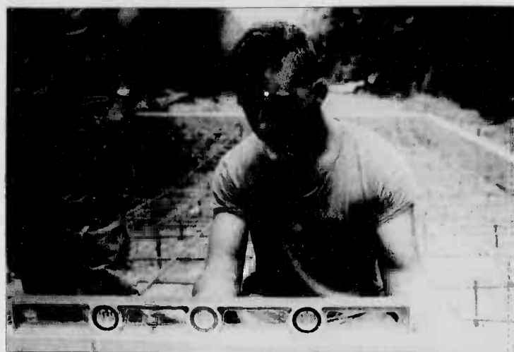
A Marine engineer ensures that the borders around a construction project are level.
