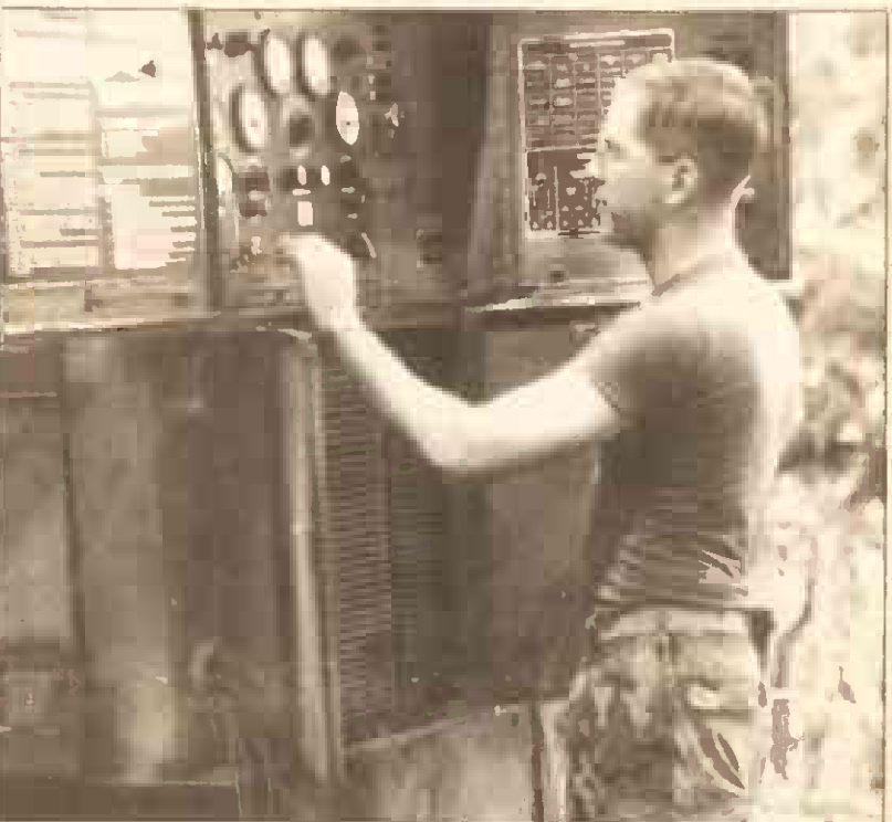
FIRE 'ER UP — Cpl. Raymond Gammon, an electrician, starts up the generator that runs the ROWPU.
