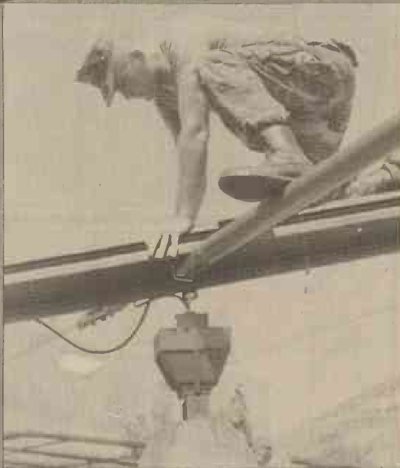
Sgt. Mark A. Wayne, project NCO, completes the installation of a light to one of the shelter's aluminum alloy beams.
