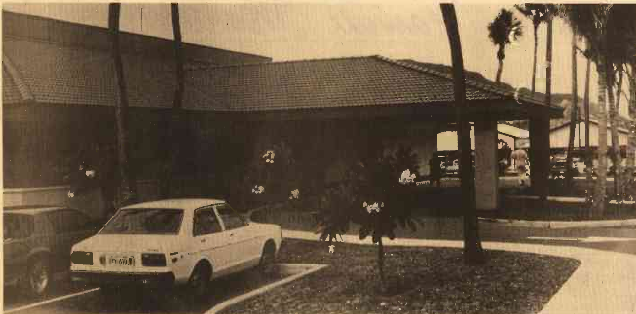
The new SNCO Club opened its doors here, July 16. The facility cost more than $2.3 million to build.
