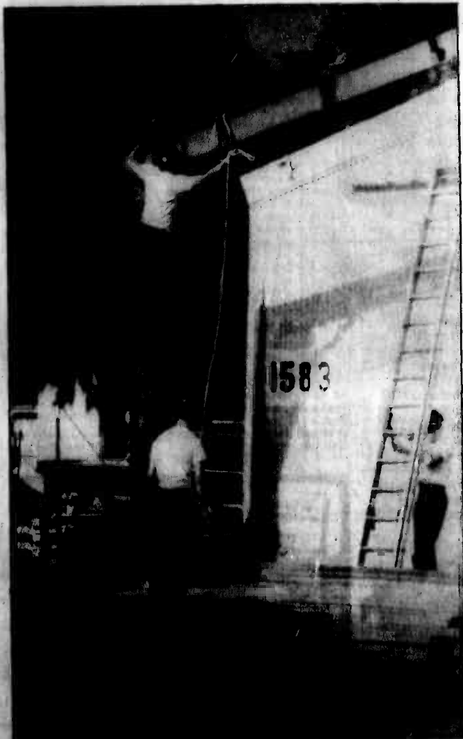
Builder 2nd Class George Bots, a Seabee reservist, ties ropes to the Station mini-gym to hold the beam in place.
