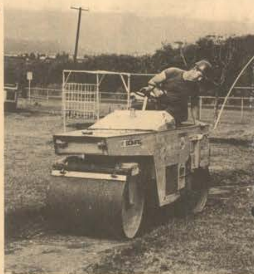
STEEL WHEEL — Equipment Operator Second Class William Boesch guides a vibrating roller along the new bicycle path at the air station's Child Care Center. Boesch, a Reserve Seabee for the past nine years, is from Hutchinson, Kan.
