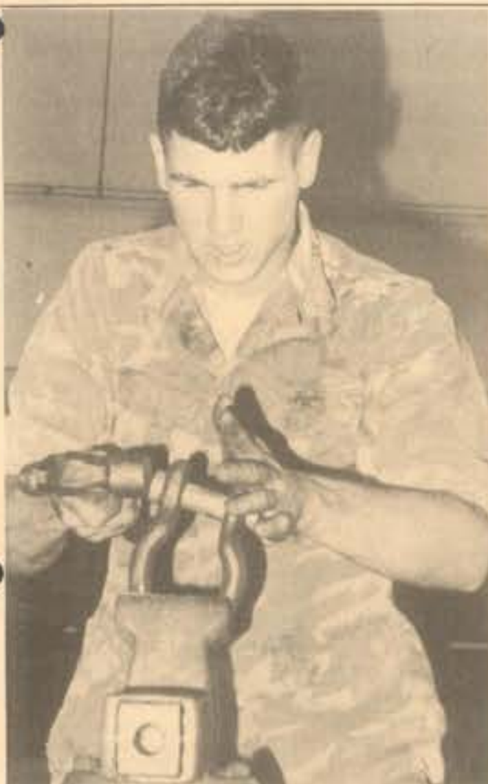
HAMMER AWAY — Private Thomas Mullin uses a hammer to fix a towing connector.
