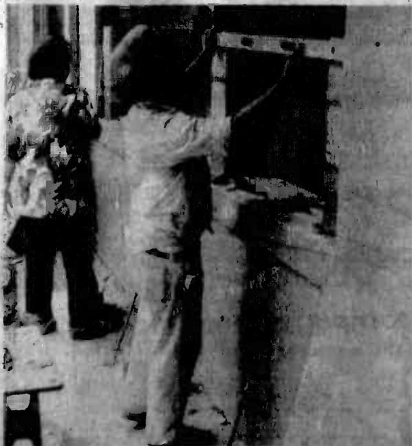
IS IT SQUARE — Carlito Corpuz, a mason, levels a window frame for the Joint Education Center classrooms as part of a remodeling project. Plans called for removing painted glass windows and replacing them with designer cement blocks.
