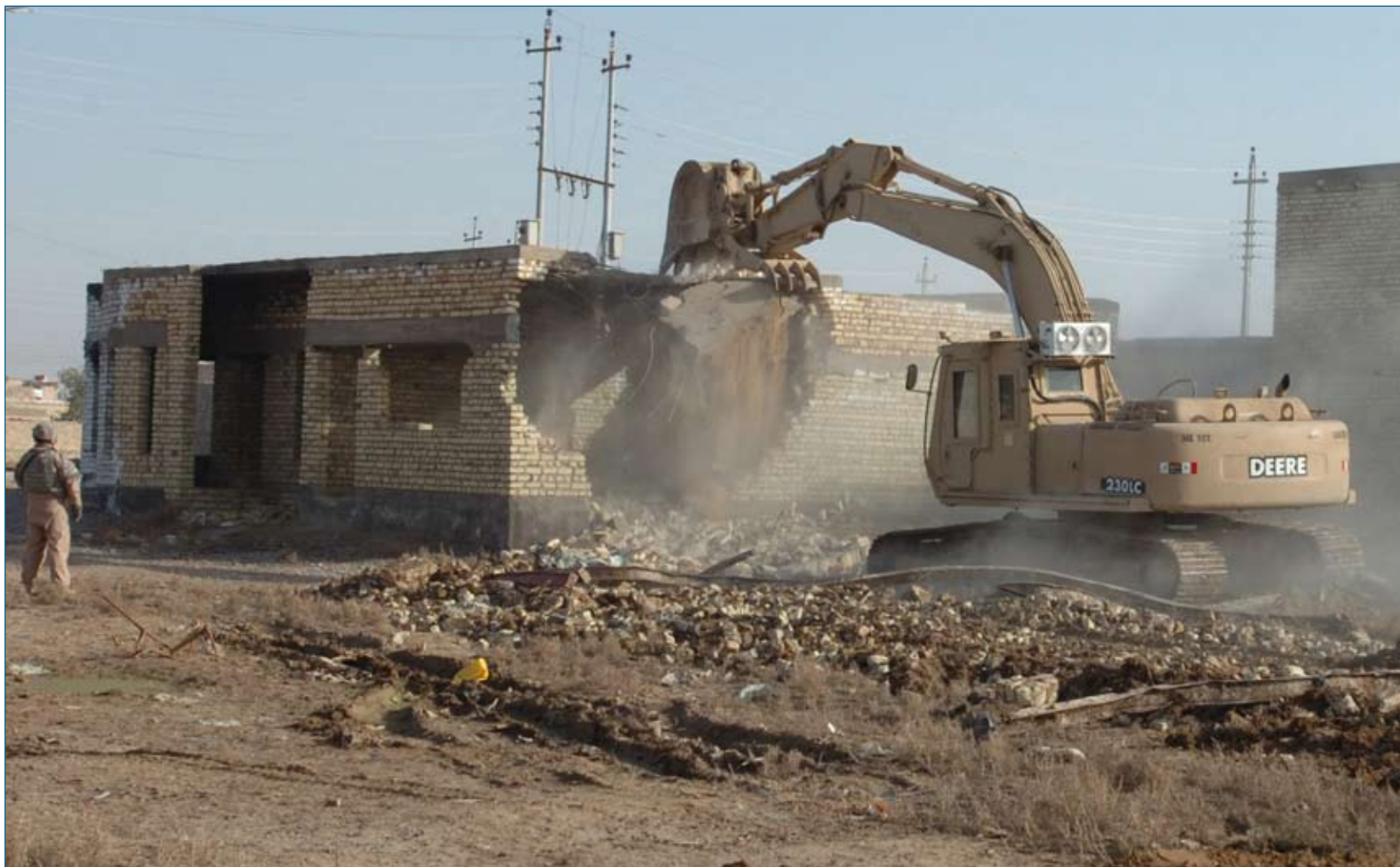
Engineers with the 92nd Engineer Battalion, assigned to the 411th Engineer Brigade, based at Logistical Support Area Anaconda, knock down the walls of an abandoned building with a back hoe
