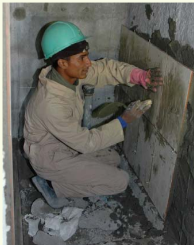
An Iraqi craftsman installs ceramic tiles in a bathroom at the project site.
