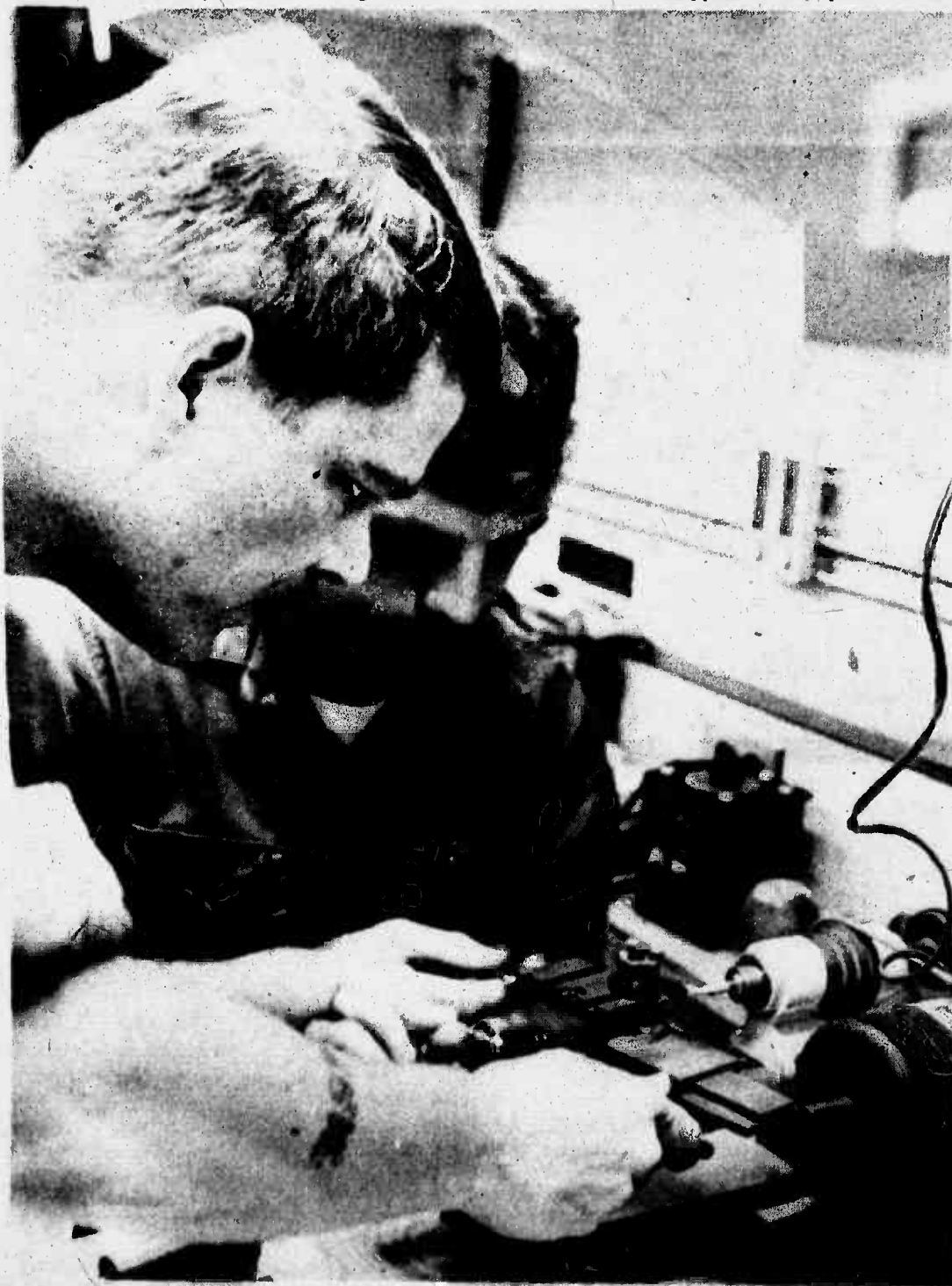
EXACTING WORK — Repairing a transistor, Staff Sergeant L.G. Buchanan (above) works late into the evening on a priority job that must be finished before he secures. Redesigning a solder iron tip (left), Buchanan helps Lance Corporal Roger Collicott (seated) set up the proper machinery. The soldering iron is one of the mini repairman's basic tools.
