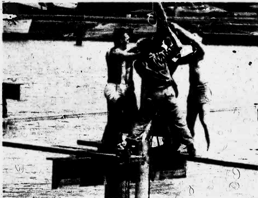
PLUG IT IN — Wiseman and I are hidden by (from left) Wight, Rose and Thompson as the five of us try to keep the rodeo bronc of a hose in the tube as it pours concrete into a submerged barrel.
