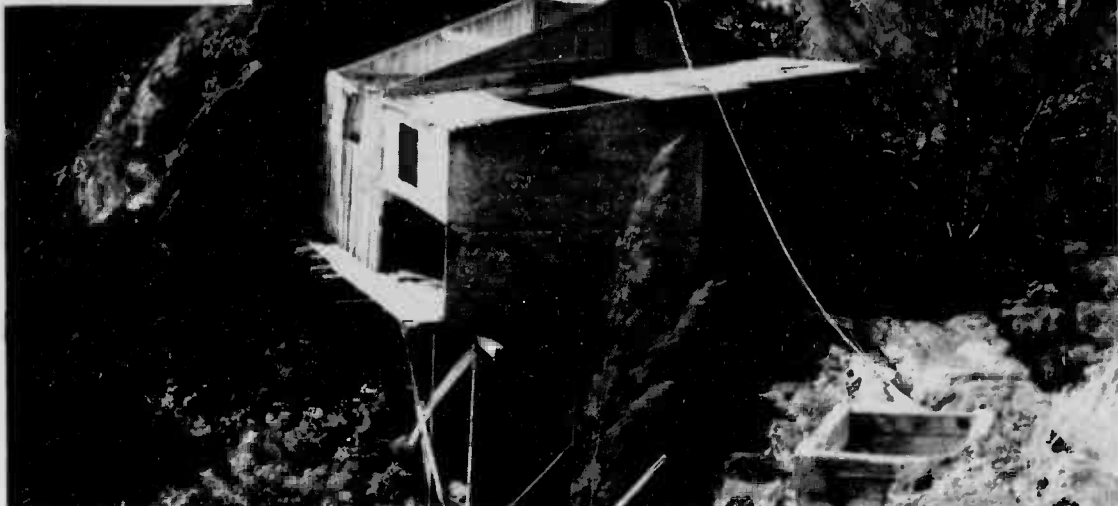
CRUMBLING - Two room wooden hut rots away in its precarious position, nestled in the crags of Ulupau Crater. The exact function of the house is not known, but it could have served as either a storage area, command post or bunking facility.
