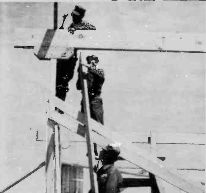
RAFTER INSTALLATION —CN J. A. Stone (l), nails a rafter in place on the new picnic shelter at Pyramid Rock Recreation Area. Assisting in the operation is (l-r): CR. R. C. Reese, and CN. Charles Del Hierro. The carpenters are members of "Seabee" Division 11-7 presently undergoing 10 days active duty training at K-Bay. The Division is scheduled to depart Aug. 31 for Santa Ana.
