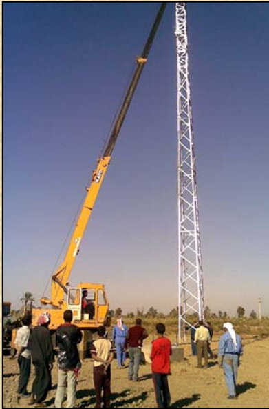
Local villagers watch as an Iraqi contractor crew sets a new electric tower in place for the Al Mazraa Tower Project in North Babil, a project to increase electrical capacity and better power transmission in the region.
