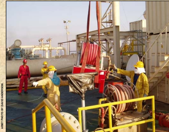
Workers lower a new hose assembly with fire-fighting foam capabilities onto the upper platform of the ABOT. Army Engineers are working several projects to increase safety and lifesaving measures.
