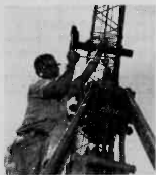
SECURES CABLE — Kenneth Tochiki, heavy duty equipment mechanic, tightens-up cable clamps on clam-shell bucket of mobile crane.
