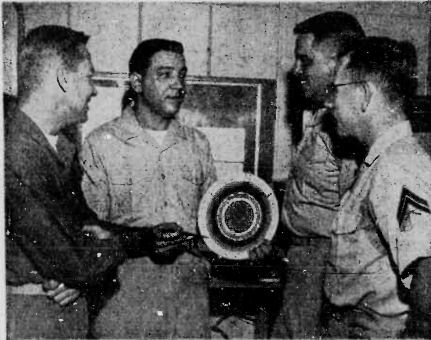
ON-THE-JOB-TRAINING — Staff Sergeant S. Krepyk, NCOIC Aerology, (center), explains use of Dew Point Computer to Sgt. T. A. Hartman, (l), to LCpl. R. J. Coe, (center right), and Cpl. D. O. Call, (r). Weathermen attend a 14-week basic course and a 22-week advanced course at Lakehurst, N. J.
