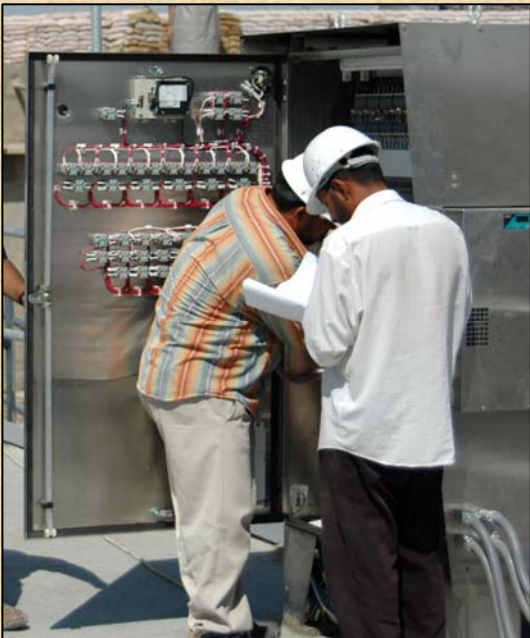
As the water treatment plant nears completion, Iraqi plant technicians will train to operate and maintain complicated systems such as the control consoles for the clarifier tanks.
