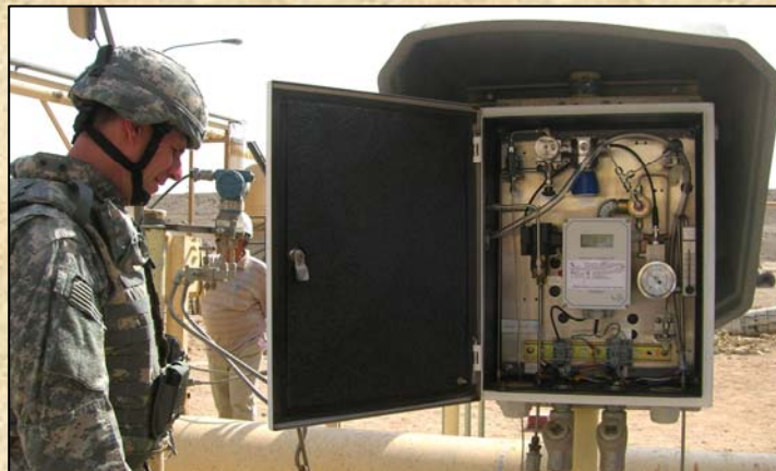
Sgt. 1st Class David Adlard with the U.S. Army Corps of Engineers checks the construction and installation of an in-line moisture analyzer at Gas Compression Station 2 near the North Rumaylah Natural Gas Liquid (NGL) plant in the Al Basrah Province, Iraq. (ARMY PHOTO)
