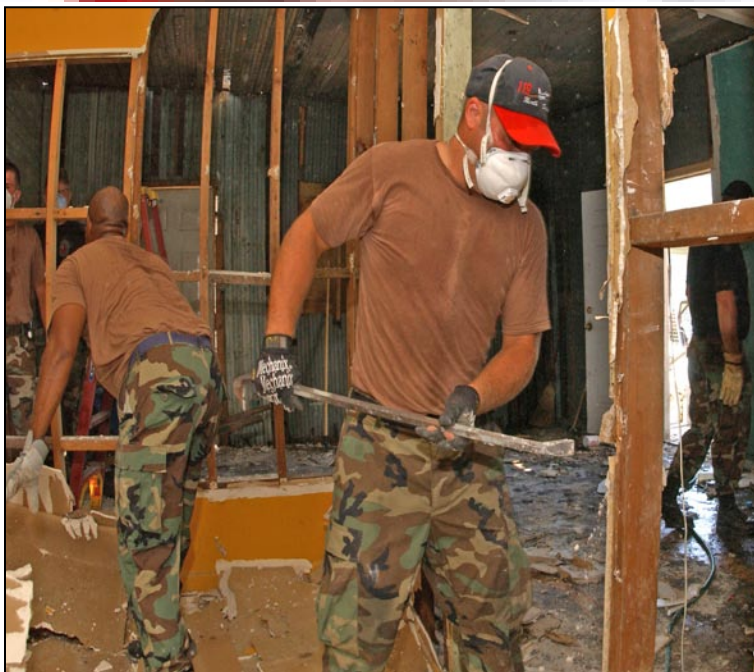
Photo by Senior Master Sgt. David Lipp, 119th Fighter Wing Senior Airman John C. Herman, 119th Fighter Wing, removes sheetrock from a Hurricane Katrina flood damaged home in D'Iberville, Miss. Sept. 14. The sheetrock must be removed because of the molds that grow on it after it was submerged in flood waters of a storm surge.
