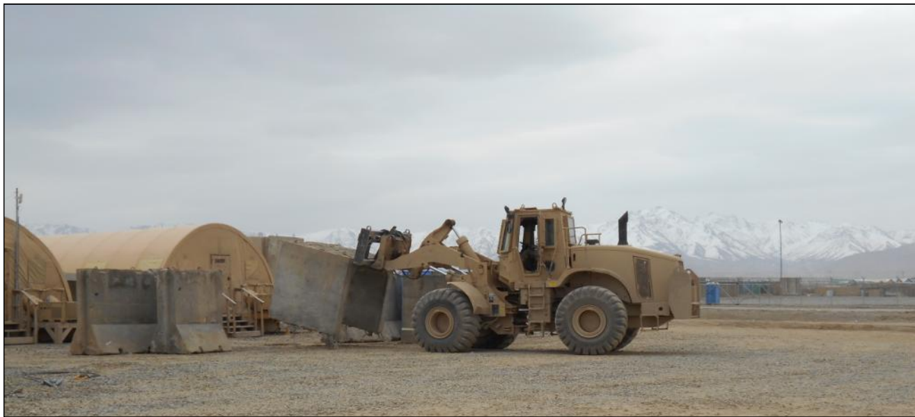
FORWARD OPERATING BASE SHANK, Afghanistan – Ennis, Texas native, Pfc. Wesley Martin, a horizontal construction engineer for the Calhoun City, Miss. - based 858th Engineer Company, attached to the Portland, Maine-based 133rd Engineer Battalion, operates a 5-yard loader to emplace a barrier at Forward Operating Base Shank, Afghanistan April 3. (Photo by 2nd Lt. John Story, 858th Engineer Company)
