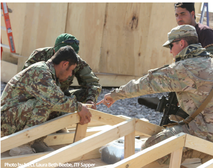
U.S. Army Spc. Steven Adams, a vertical engineer with the 284th Eng. Company, explains to some Afghan National Army soldiers with the 207th CEK how to construct trusses for a roof they were assembling for a guard shack at Camp Zafar, Western Afghanistan.
