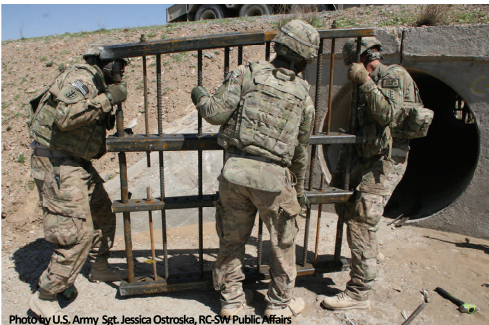
Soldiers with the 82nd Eng. Co. install a culvert denial system along Hwy 1, designed to prevent the emplacement of IEDs in small tunnels along the highway and ensure the safety of the travelers on the road.
