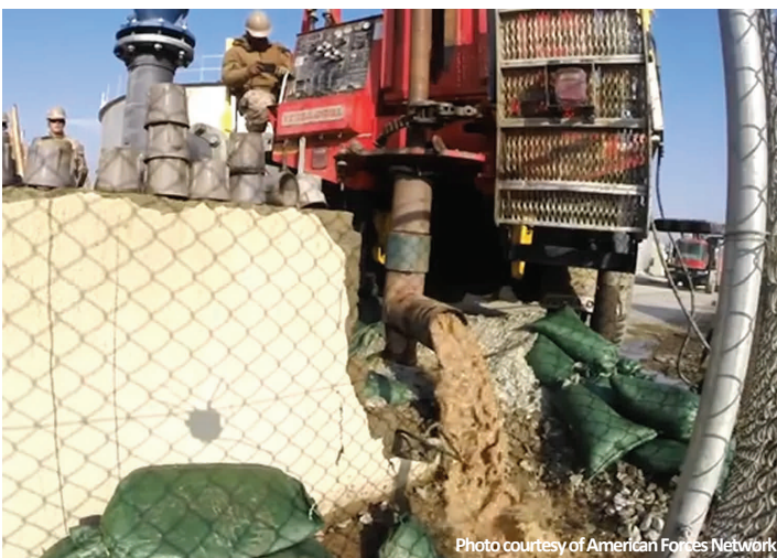
A diverter is used to force the water from the well into a specific direction the Seabees want it to go after being forced through the filters
