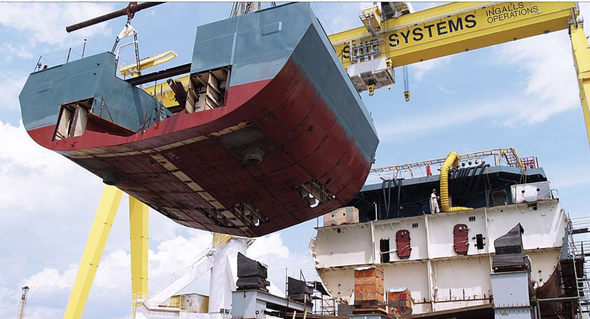
↑ STERN LAUNCH The stern assembly is placed onto the second National Security Cutter, CGC Waesche, in Pascagoula, Miss., Sept. 11, 2007. The placement of the stern marks the 34th unit fitted onto the Waesche, completing 33-percent of the ship.
