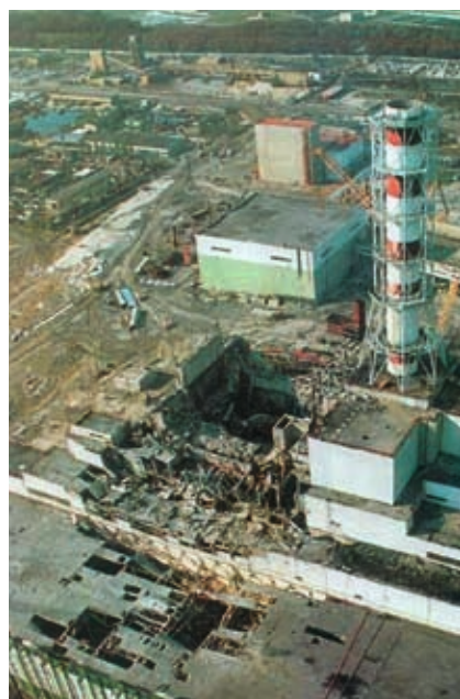
Chernobyl reactor number four after the disaster, showing the extensive damage to the main reactor hall (image centre) and turbine building (image lower left).
