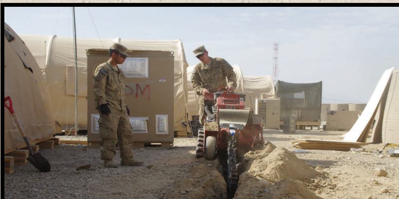
Communication is very important for all the companies. Here, 84th Soldiers are digging a small trench for commo lines to be laid.
