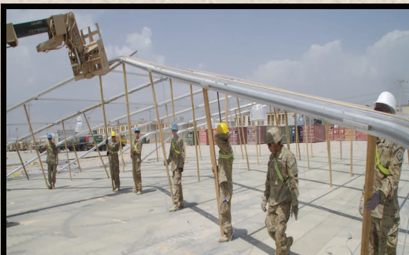
In addition to deconstruction, the battalion has also been constructed multiple projects. In order to help the retrograding process, 585th built two LAMS-A tents that will later be used as storage and holding areas for CMRE sorting
