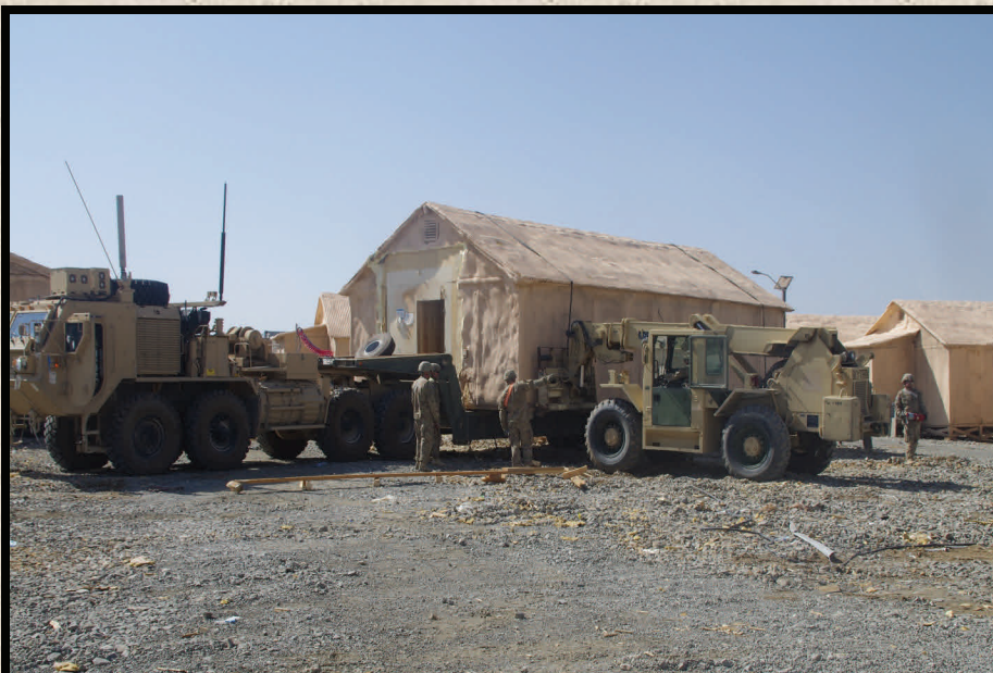
1220th Engineer Company Soldiers discovered a faster way to deconstruct small structures: move it as a whole instead of taking it apart piece by piece.
