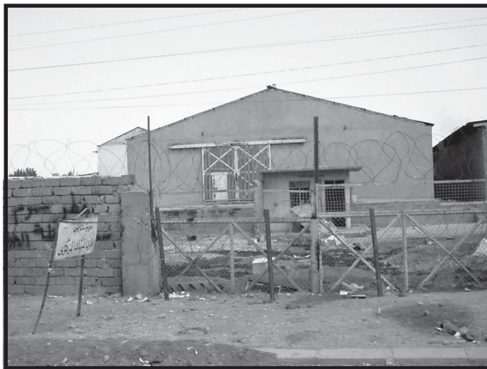
The agricultural warehouse, decontaminated and secured
