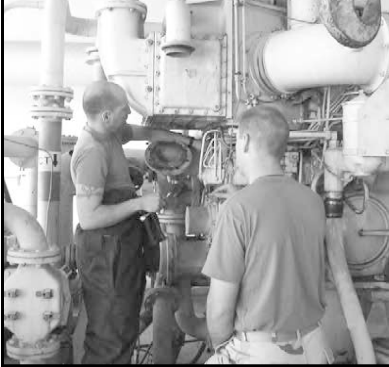
Two prime-power soldiers repair an Iraqi generator.
