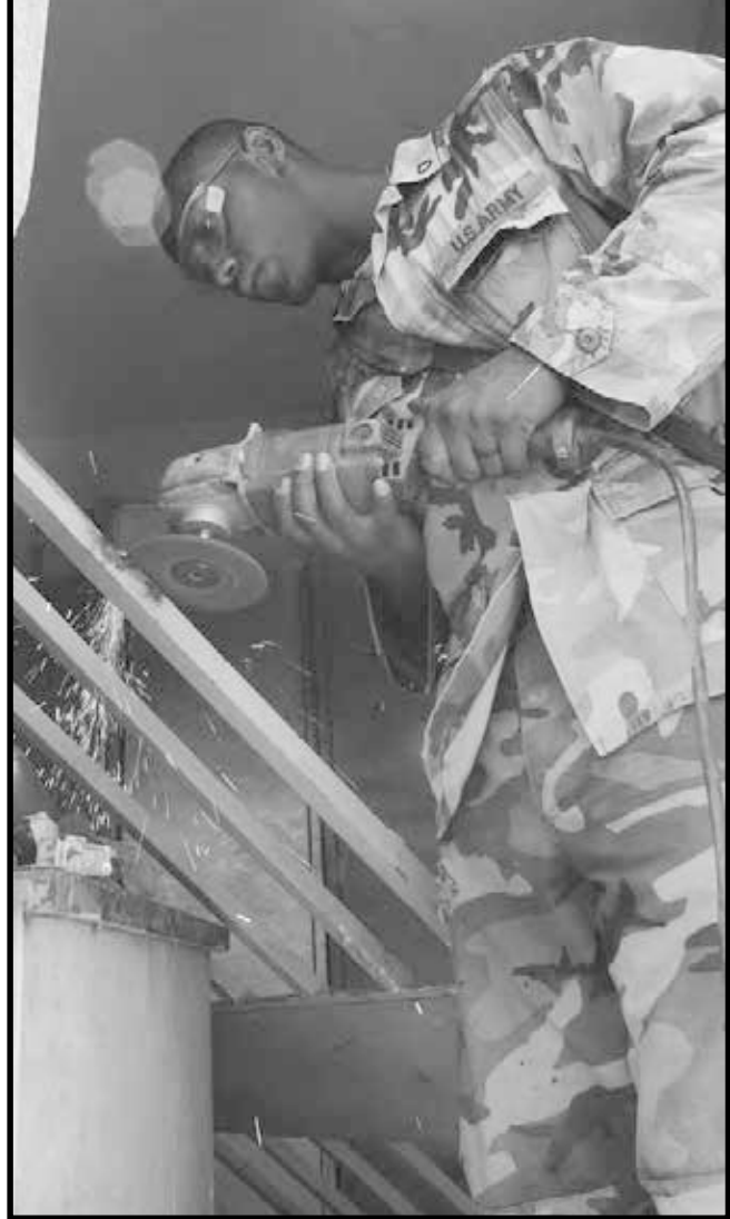
A metalworker with the 535th Engineer Company braces a steel door while grinding off the rough spots. Soldiers welded hinges and repaired doors at an elementary school in Al Hurriyah, Baghdad.
