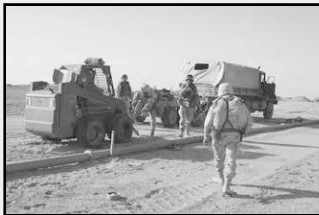
The battalion's Bobcats were invaluable in constructing the pipeline.
