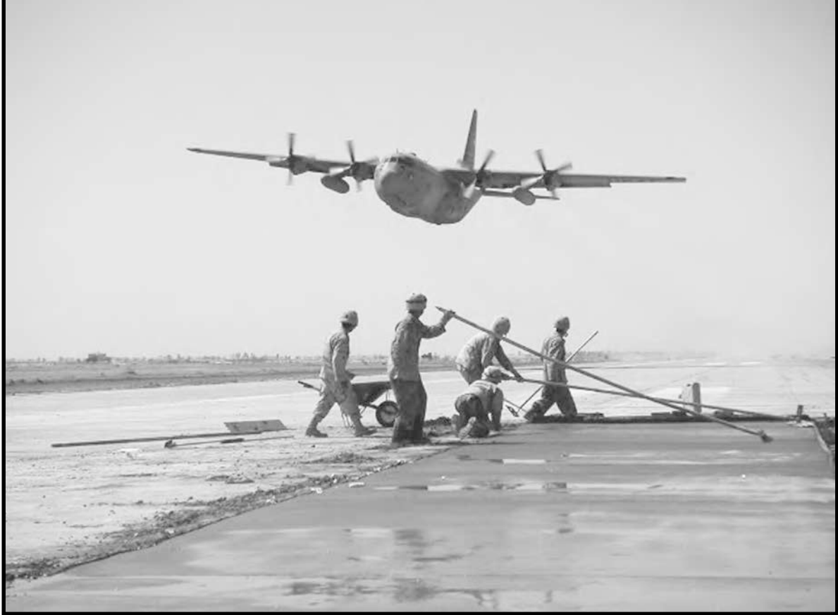
Engineer soldiers repair the airfield at LSA Anaconda, near Balad, Iraq.
