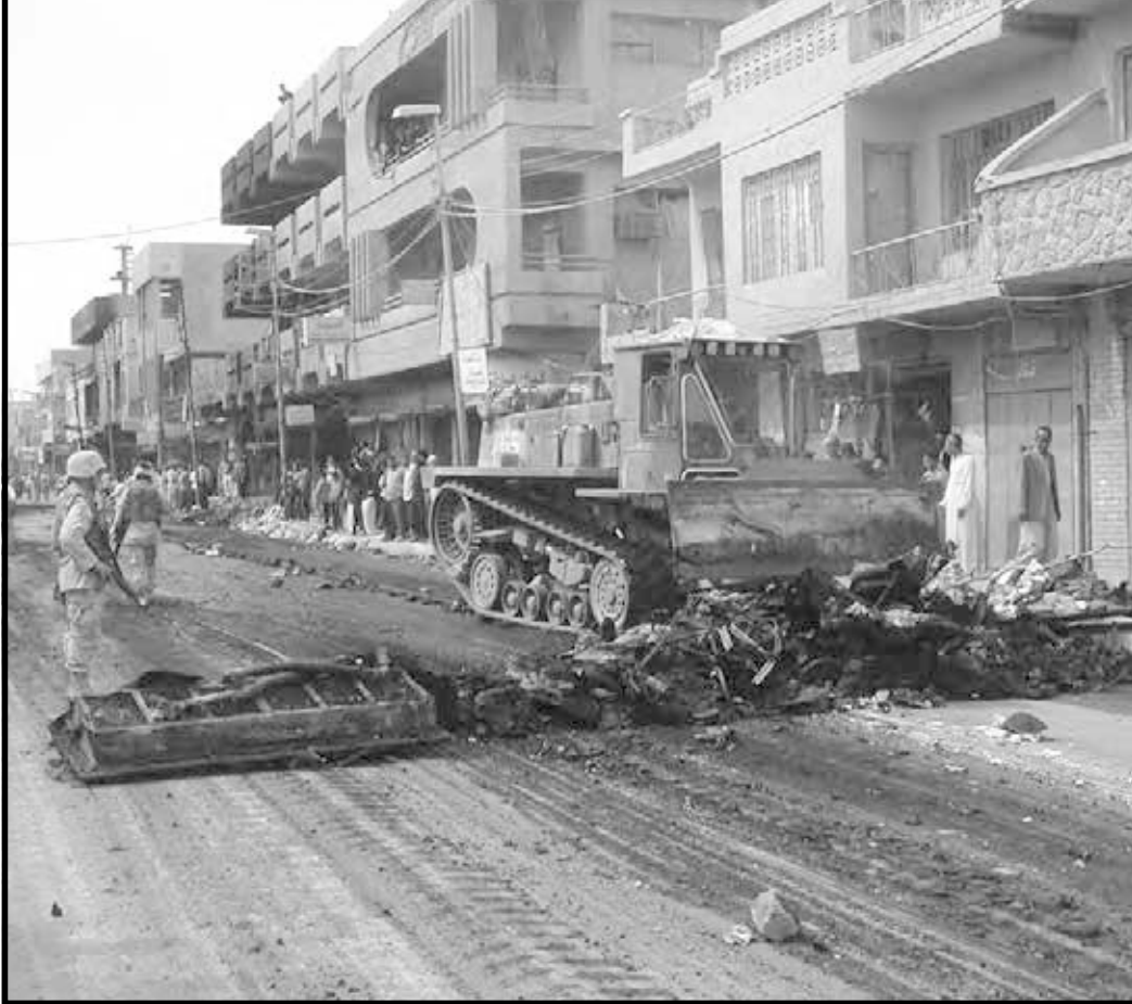
The 887th Engineer Company clears battlefield debris (destroyed T-72s) using the company's DEUCes in the town of Al Mahmadiyah, Iraq, south of Baghdad.
