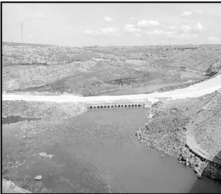
A 6,700-foot heavy equipment transport bypass for Seyhvelet Bridge
