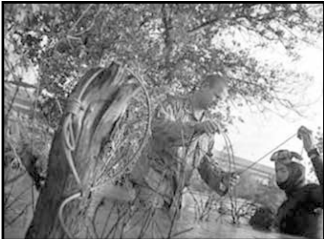
Divers emplace detonation cord in preparation for clearing underwater obstacles.
