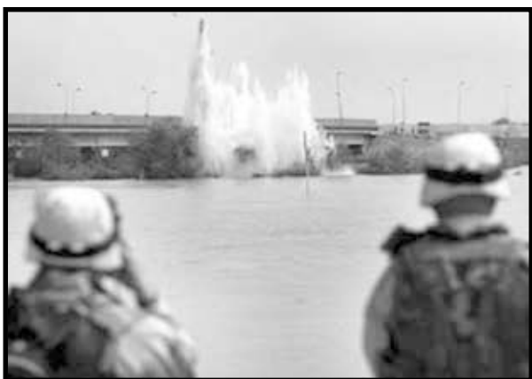
Divers from the 74th Engineer Team (Dive) stand on the shore as they watch a bridge blow after a demolition emplacement mission.
