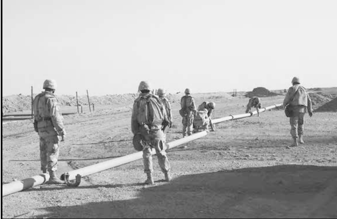
Engineers lay pipe for the IPDS.
