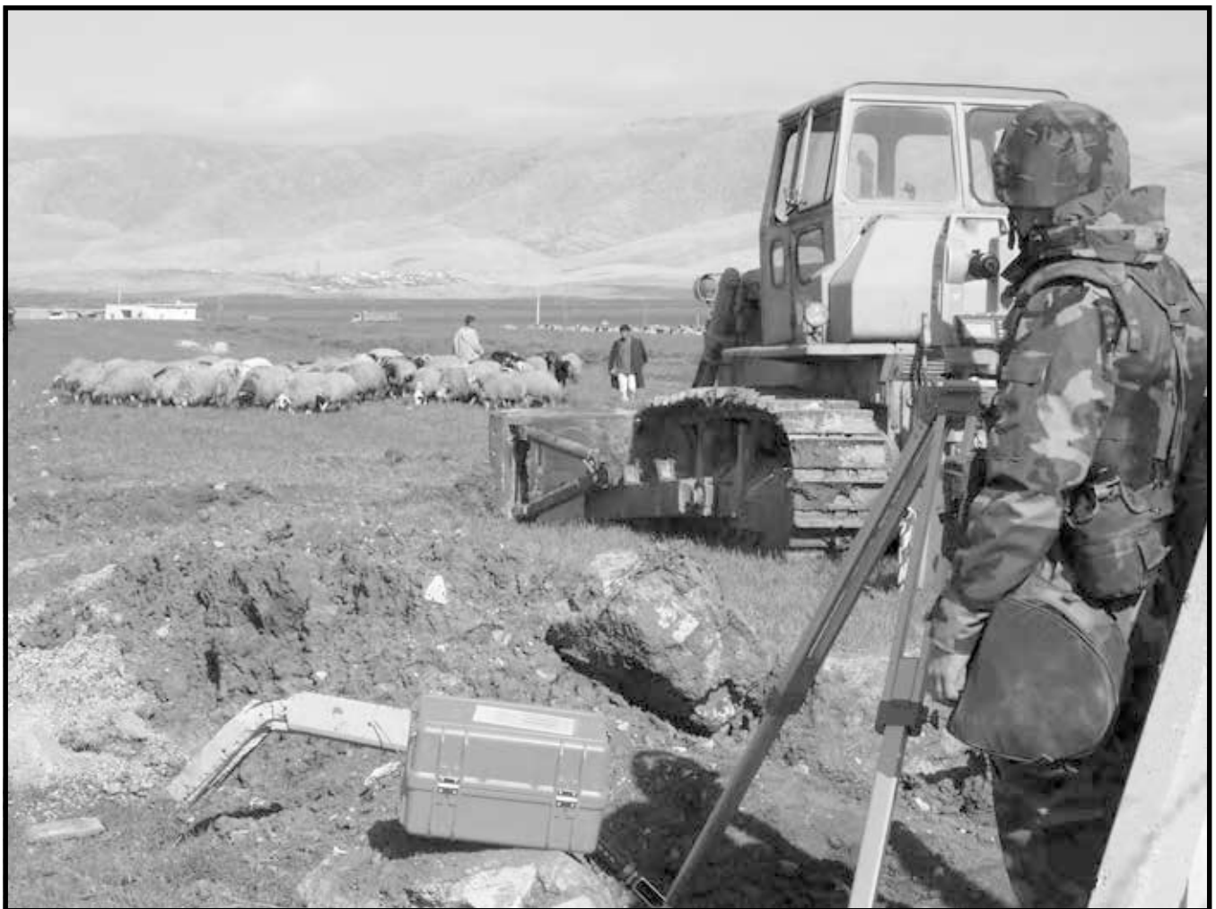
A Seabee from Naval Mobile Construction Battalion 4 surveys for the logistics support area near Nusaybin, Turkey.
