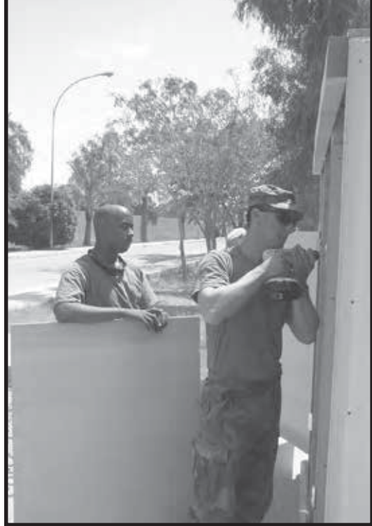
Soldiers construct a latrine at Ar Ramadi, west of al Fallujah.
