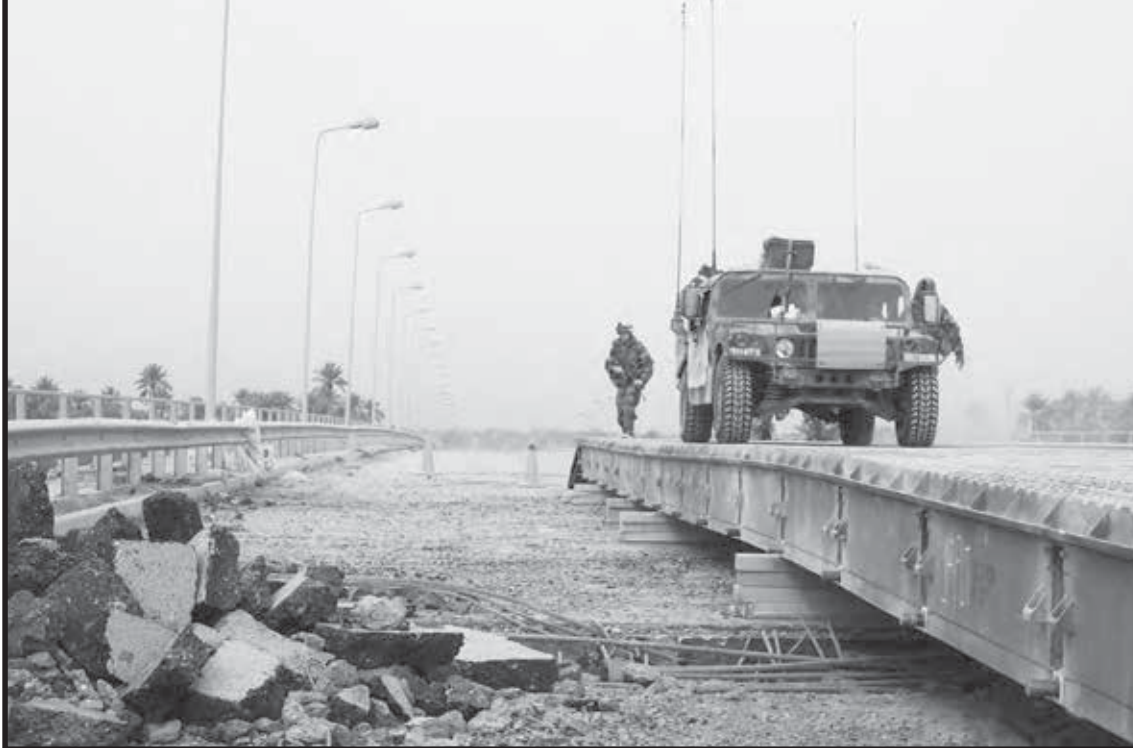
A HMMWV crosses a newly completed medium girder bridge at Objective Peach.
