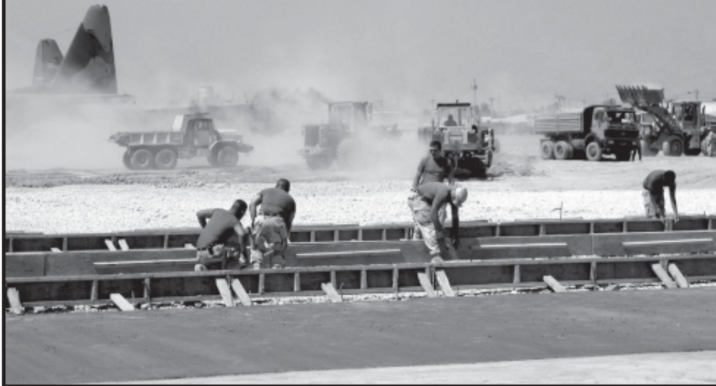
Soldiers of Task Force Coyote construct concrete forms in preparation for placement of concrete to increase aircraft parking space at Bagram Airfield. In the background, the dust flies as crews work ahead of the concrete placement group.
