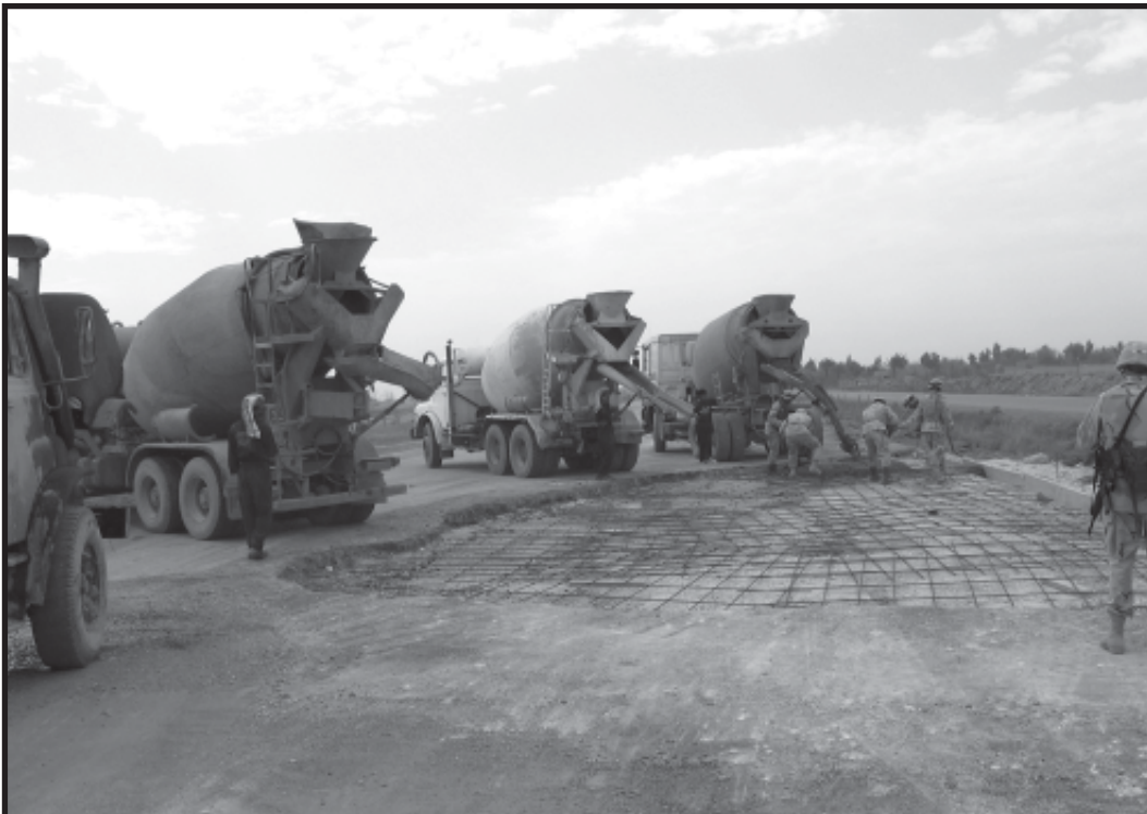
A local contractor provided the concrete that Task Force Black Diamonds placed to repair Crater B.
