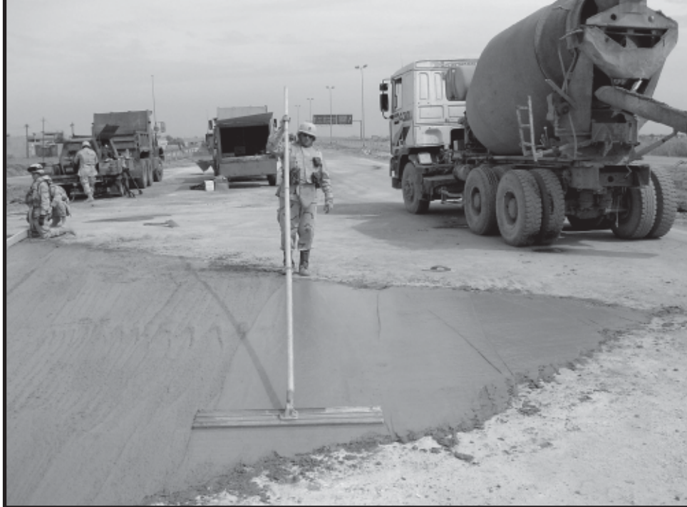
A Task Force Black Diamonds Soldier uses a float to finish the repair of a crater after the vibrating and screeding process.
