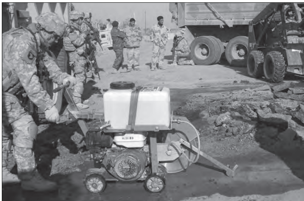
535th ESC Soldiers repair an IED crater.
