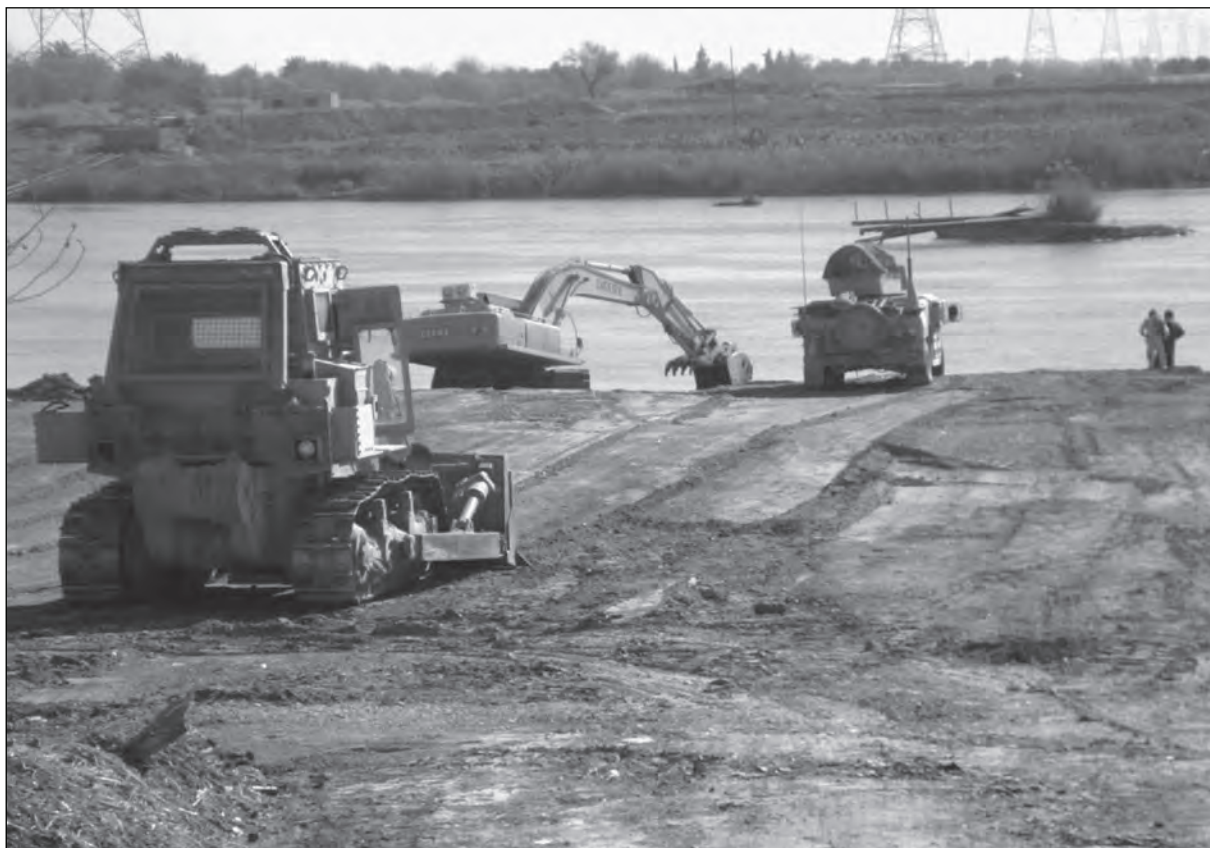
535th ESC Soldiers prepare the approach for an assault float bridge.
