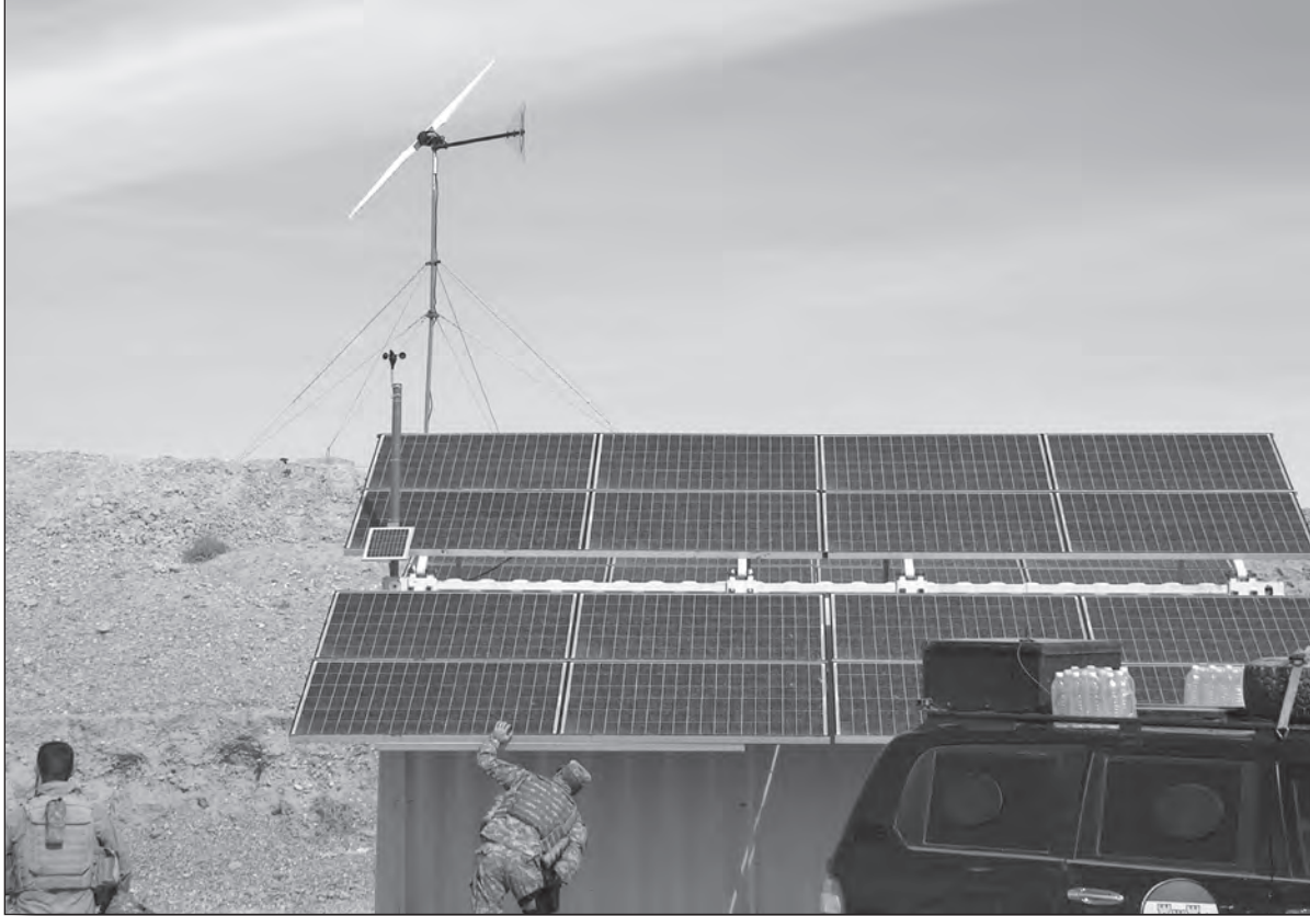
MNSTC-I inspection of solar panels and wind turbine
