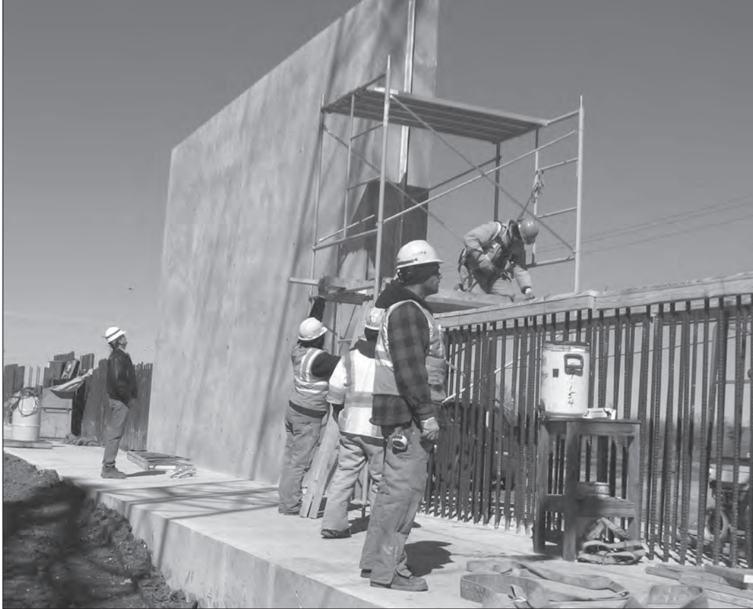
New Orleans West Bank floodwall—part of Task Force Hope’s risk-reduction efforts
